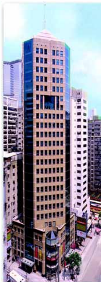
Chuang's Enterprises Building
