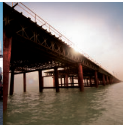
Yellow Sea Crossing-linking the man-made island and industrial and logistics park 連接人工島及工業物流園的黃海大橋
