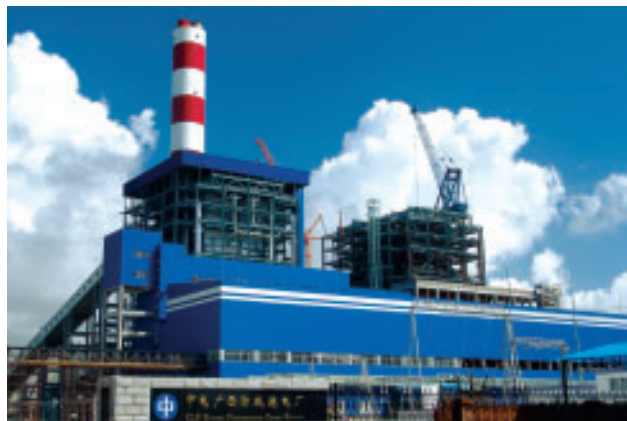
Fangchenggang project – nearing commissioning
