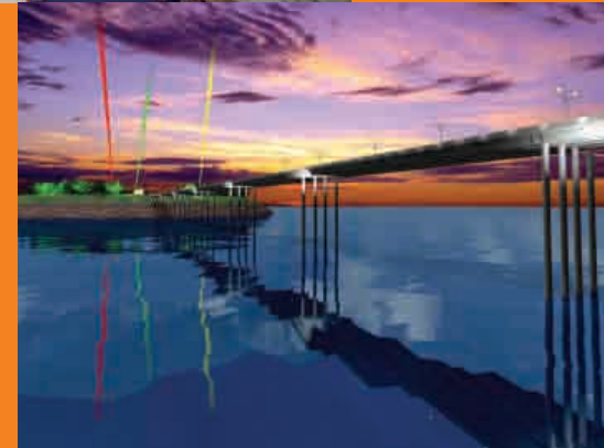
Hong Kong-Zhuhai-Macau Bridge Project (proposed by Hopewell)
