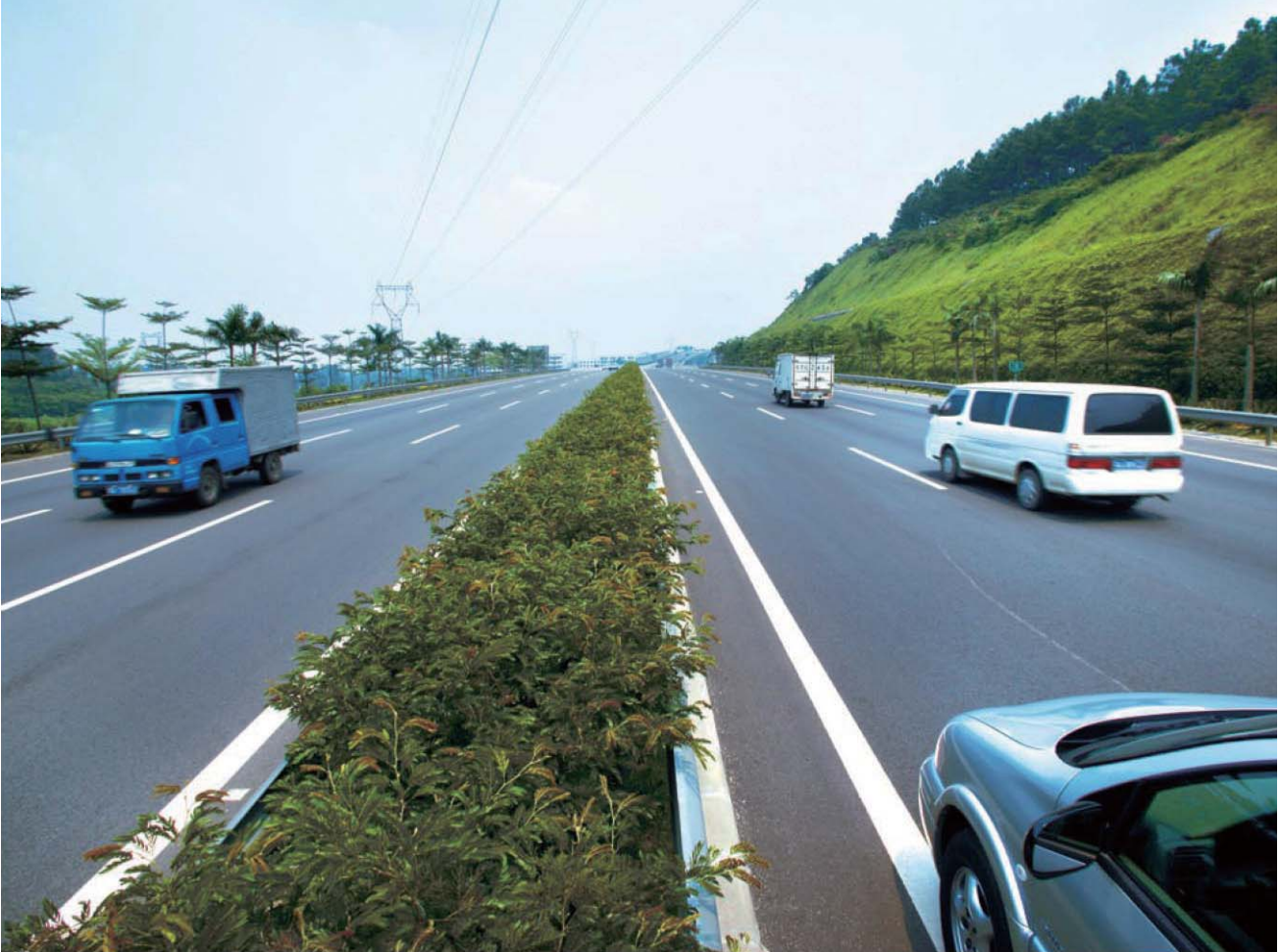
Phase I West
