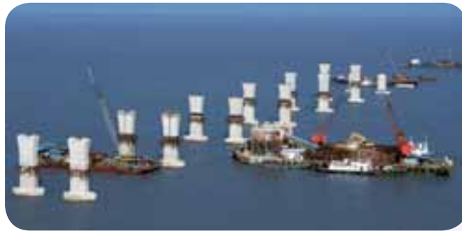
Installation of precast tower pillars
