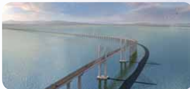
Nan'ao Bridge in Guangdong Province (artistic illustration)
