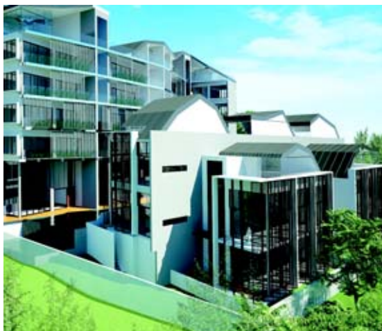
Aura Park, property development project in Singapore
