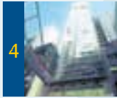
4 235 Wing Lok Street Trade Centre Property Sheung Wan, 52,285 sq.ft.
