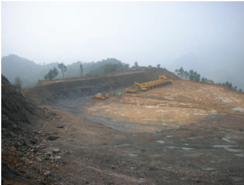
Figure 6-4: Jinfeng Mining Equipment
