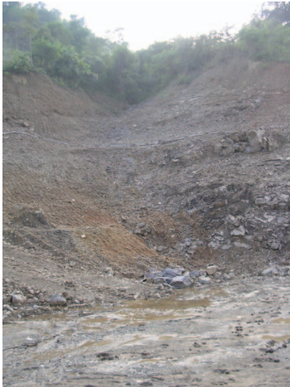
Figure 5-27: CIL Embankment Construction, 15 October 2006
