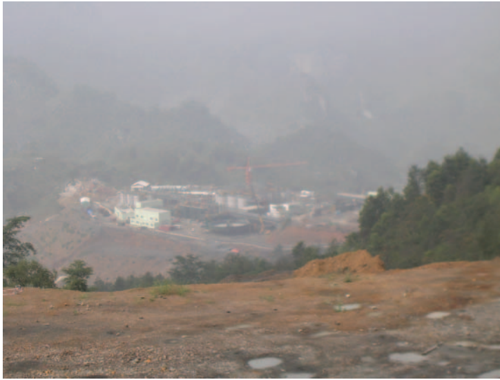
Figure 5-29: Photograph Showing General Plant Layout, 15 October 2006
