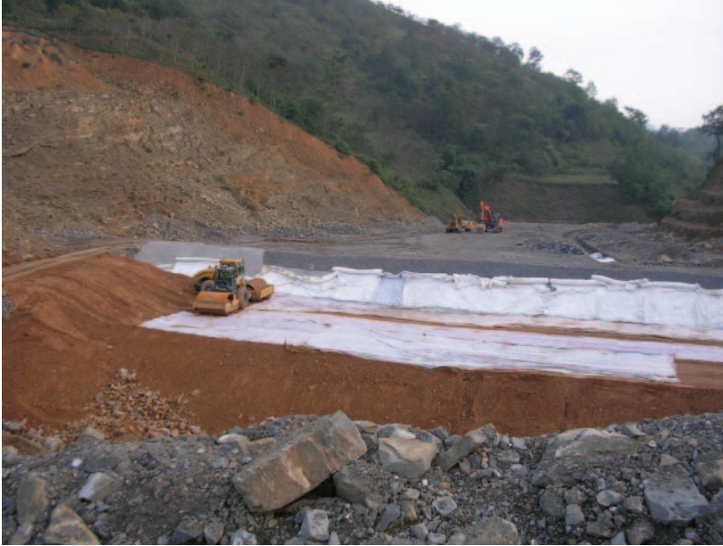
Figure 5-22: Construction of Flotation TSF Embankment, October 2006
