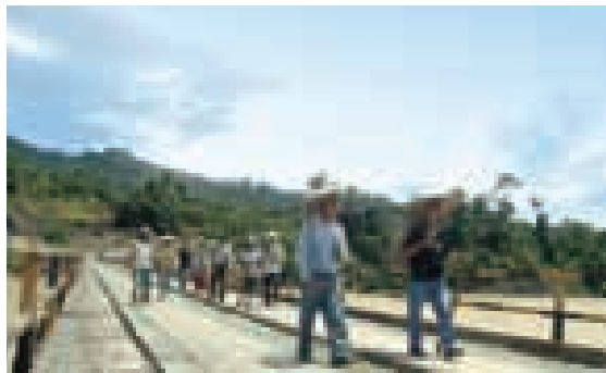
Over the years, the Group's road network and bridges have provided much needed access to the local communities within the forest through safer and more convenient routes.
