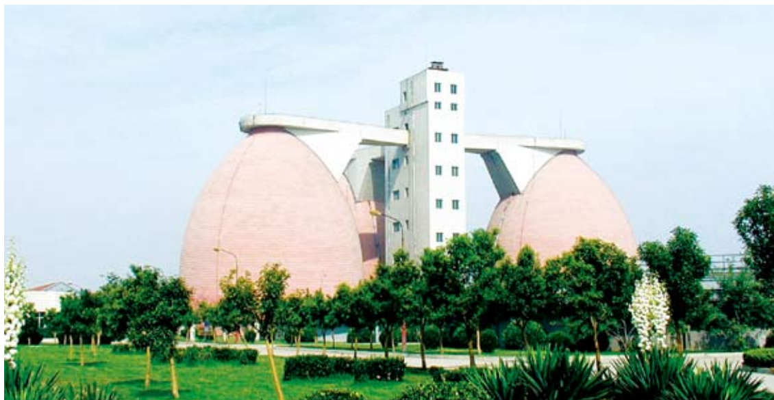
Jinan Waste Water Treatment Plant 濟南污水處理廠
