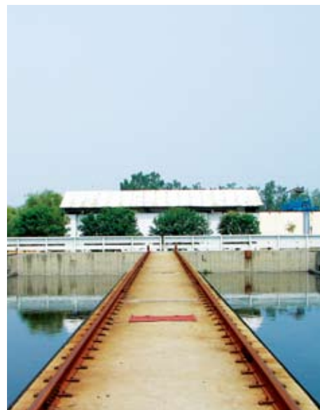
Qingdao Haibohe Waste Water Treatment Plant 青島海泊河污水處理廠
