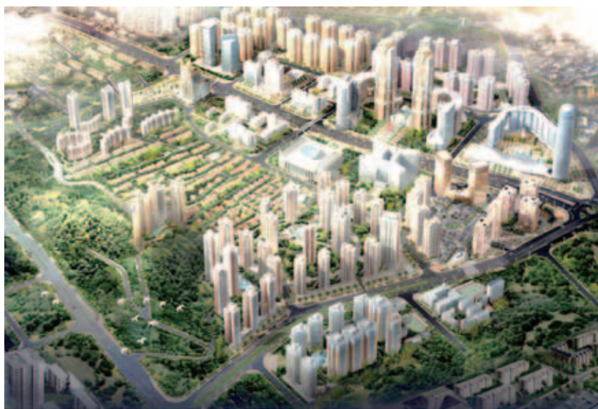
Main Land Bank in Chongqing
