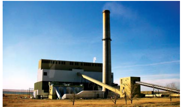
This coal-fired power plant in Sheerness, Alberta, is one of six power plants included in the Stanley Power Inc. transaction.
