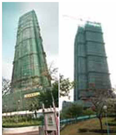
83 Sycamore Street 6 Cho Yuen Street
