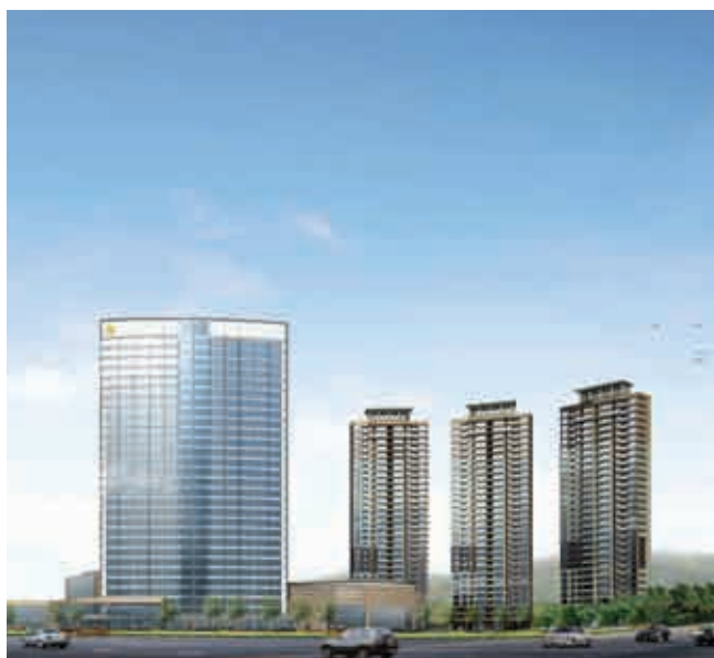
Yangzhou hotel and apartment project, Yangzhou, MAINLAND CHINA*
