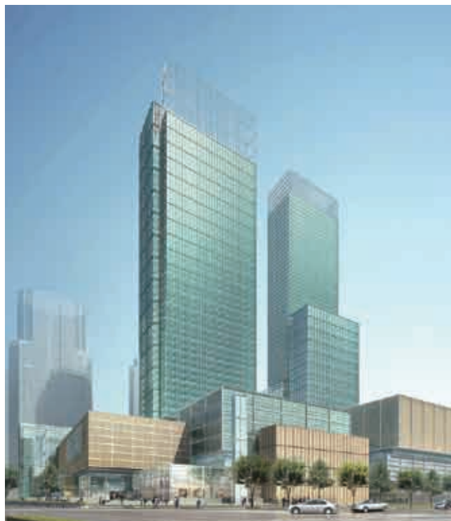
Jing An Kerry Centre, Shanghai, MAINLAND CHINA*
