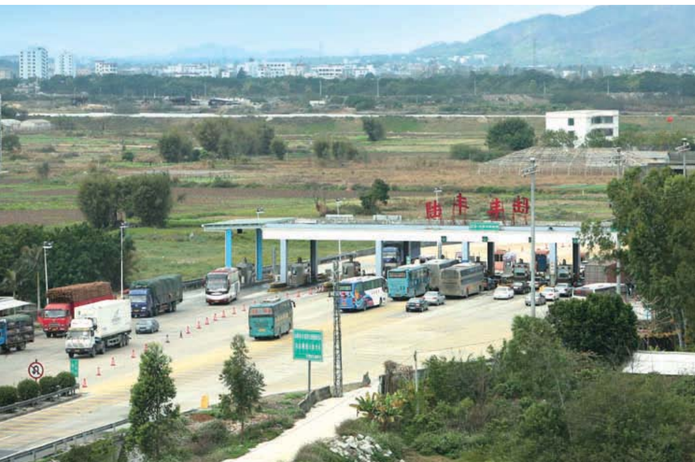
The Shen-Shan Highway (Eastern Section) recorded double-digit growth in toll revenue during the year.
