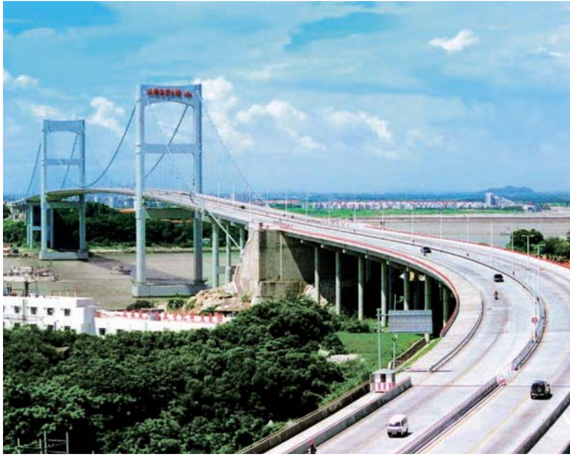
Boosted by strong growth in Guangdong Province, Shantou Bay Bridge performed well in 2007.
