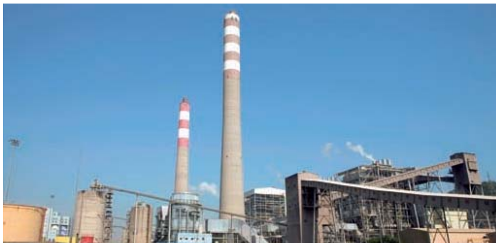
As an extension to the Zhuhai Power Plant, Jinwan Phase 1 Power Plant project was commissioned and has provided profit contribution since February 2007.
