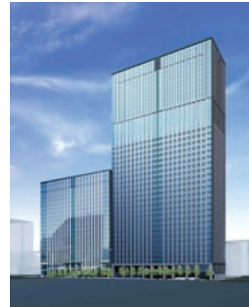
2009 Shangri-La Hotel, Tokyo
