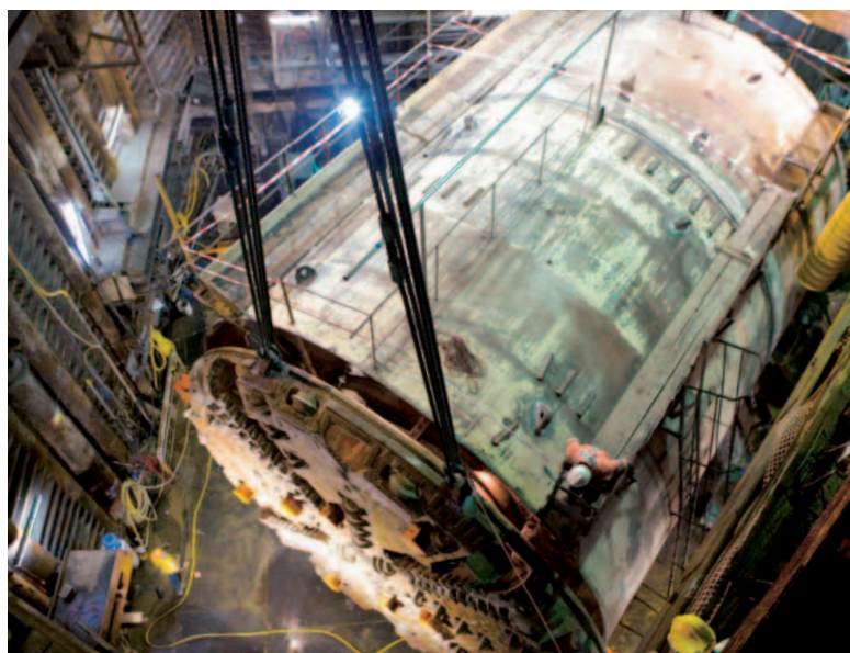
Construction works on the Kowloon Southern Link
