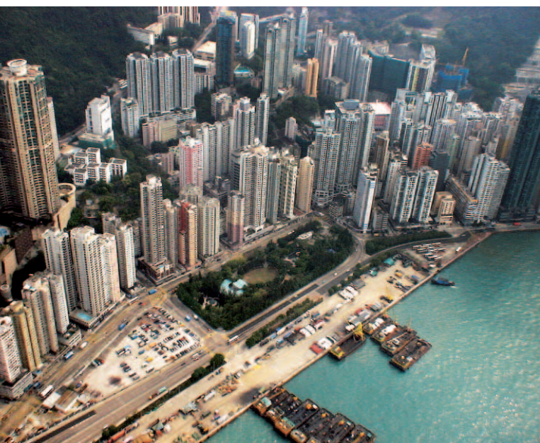
The proposed West Island Line is an extension of the Island Line
