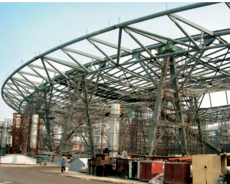
Steady progress was made on the Beijing Metro Line 4 (BJL4) project
