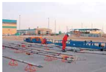
ELIS logging system operated in the United Arab Emirates
