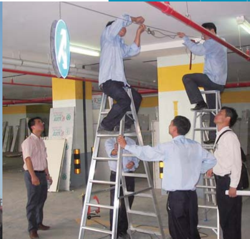
Engineers of Comba working on-site
