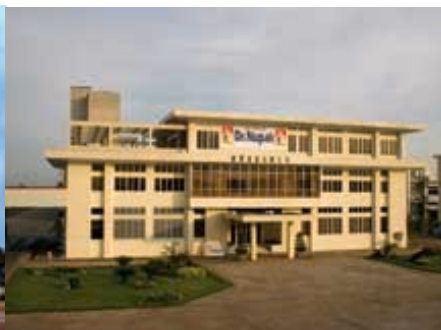
Asia Nutrition Technologies (HN) Co., Ltd. Feed production plant in Hanoi, Vietnam
