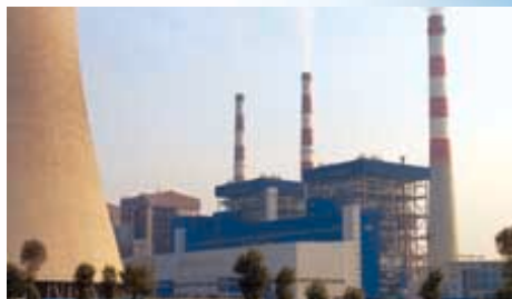
Pingwei Power Plant II
