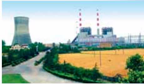
Pingwei Power Plant
