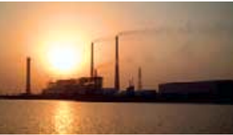
Changshu Power Plant
