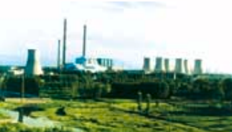
Shentou I Power Plant
