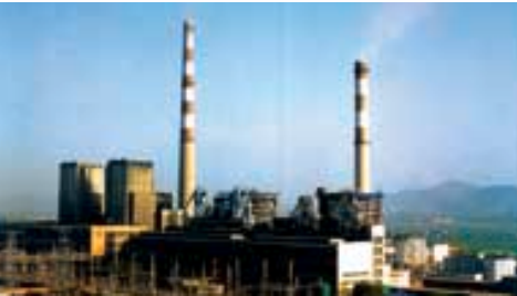
Yaomeng Power Plant
