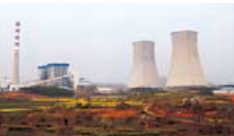
Huanggang Dabieshan Power Plant
