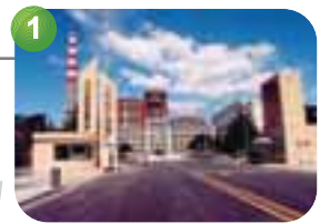
Gao Jing Thermal Power Plant
