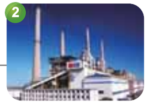
Dou He Power Plant
