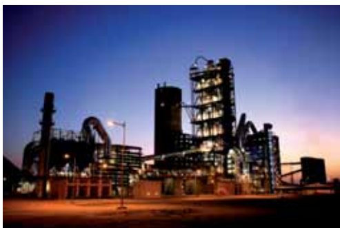
RCC 5,000TPD cement production line, Saudi Arabia
