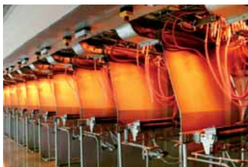
Alkali-free direct-melt glass fiber production line
