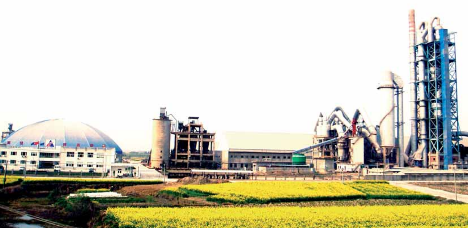
5,000TPD Clinker production line, Tianshan Cement
