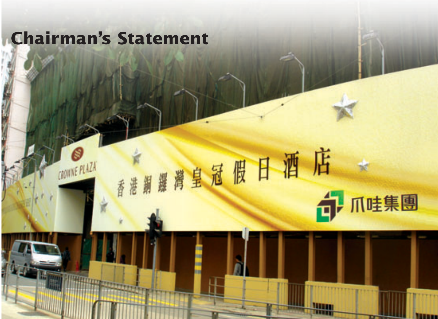
Superstructure works of Crowne Plaza Hong Kong Causeway Bay
