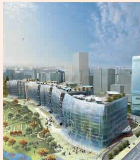
Above is an artist's rendition of the Shanghai Gaoyang International Passenger Transport Centre
