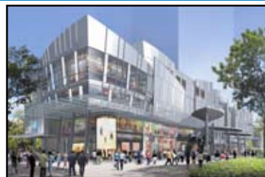
New Mandarin Gallery, an OUE property project in Singapore
