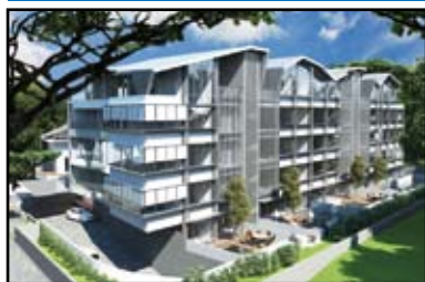
Aura Park, property development project in Singapore
