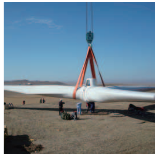
◀ 4. Preparing to install the blades
