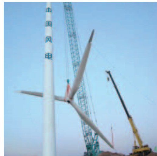
◀ 5. Lifting the blades
