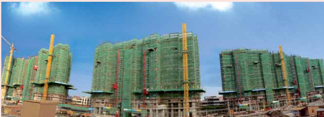
Imperial Garden – perspective (above); under construction (below)
