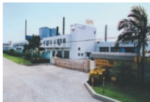
Front View of the Industrial Laminate Plant in Zhongshan, the PRC
