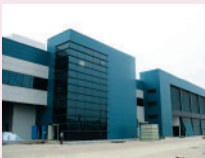
廠房正面(建築面積30,373 m 2 ) Factory-front (Gross Area 30,373 m 2 )
