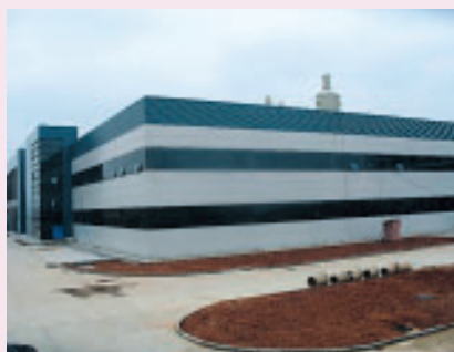
廠房側面 Factory-side
