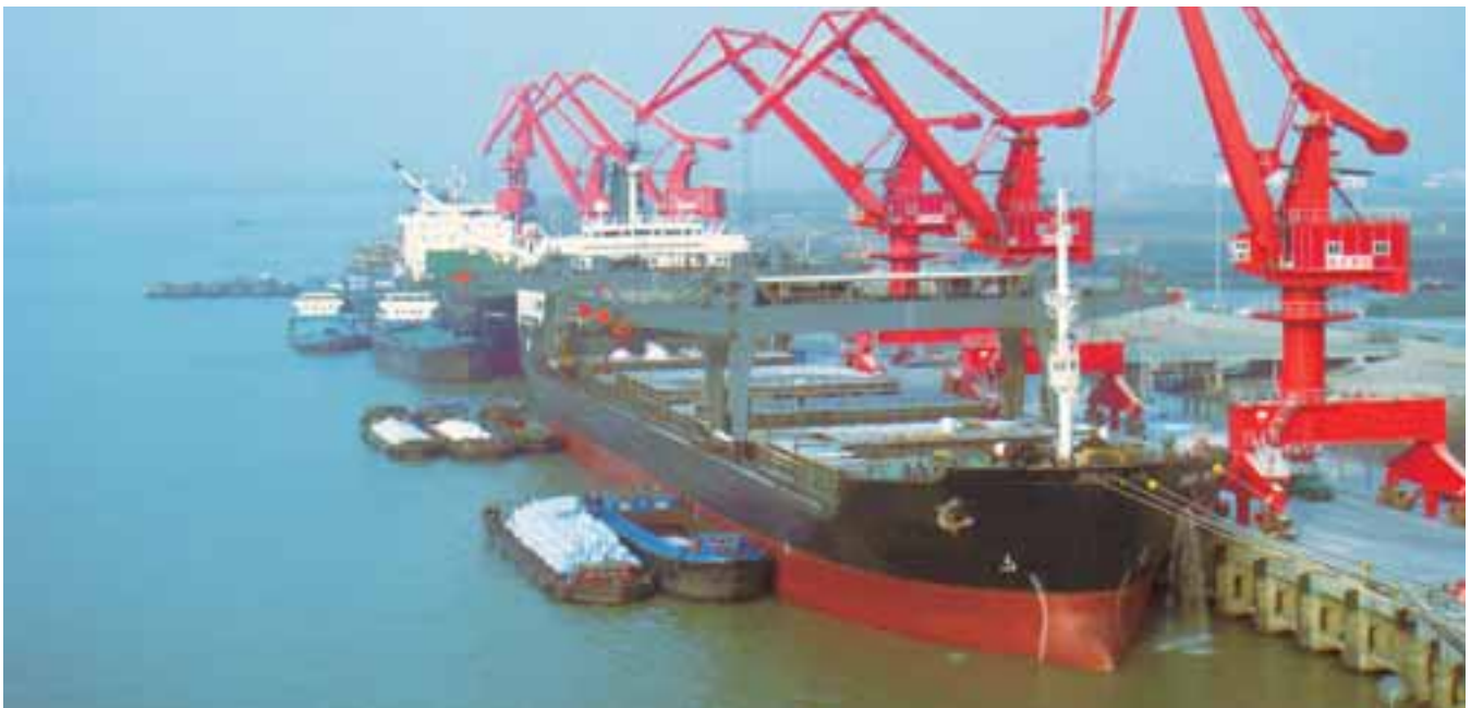
Nanjing Longtan Tianyu Terminal
