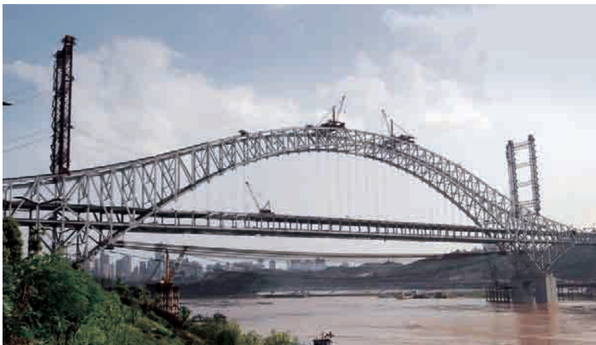
(Chongqing Chaotianmen Yangtze River Bridge, The main body of the bridge is 1,741 metres long. A steel truss girder tier-bar arch bridge with the longest span in the world of its type.)
