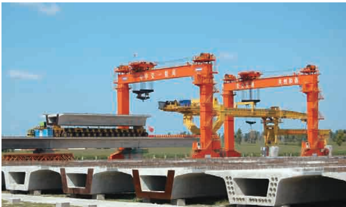
(Harbin-Dalian PDL, the first girder casting ceremony).
