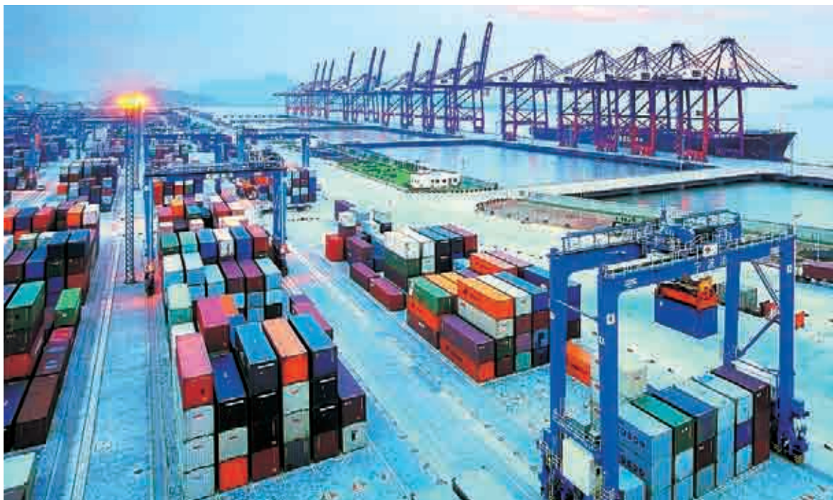
(Phase IV and V of Beilun Container Terminal project of Ningbo Port, totalling 10 berths accommodating over 10,000 DWT with throughput capacity of 10 million TEUs by 2010.)
