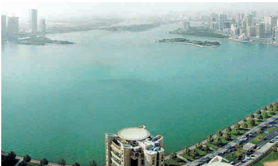
(Khalid Lagoon Edge Wall-Sharjah project in UAE. Phase II of Khalid Lagoon edge Wall-Sharjah project is an important component of coastal line extension program, which receives a great deal of attention from the local government.)
