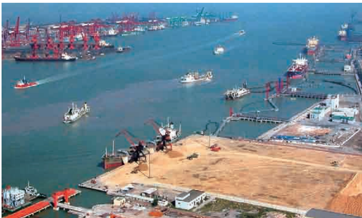
(Phase I of Channel Expansion Project of Tianjin Port, with an engineering capacity of 9,150,000 cubic metres to accommodate the navigation of vessels of 150,000 to 200,000 DWT.)
