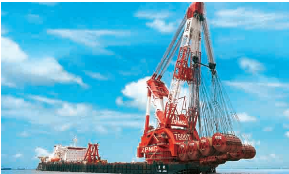
("Lan Jing" — 7,500 tons full-rotary floating crane with lifting capacity of 7,500 tons. It is the largest craning vessel in the world which is researched and developed by China with qualification certificate of navigation worldwide.)
