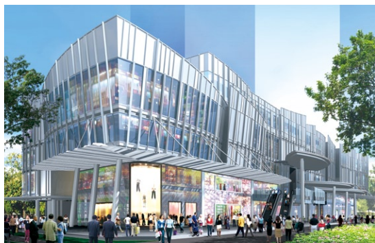
New Mandarin Gallery, an OUE property project in Singapore
