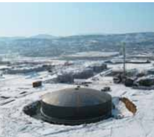
▲ The natural gas liquefaction plant taking shape in Shanxi.
