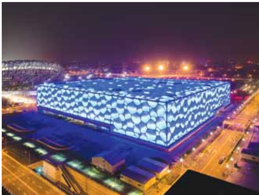
▲ The National Aquatic Centre “Water Cube” in Beijing
