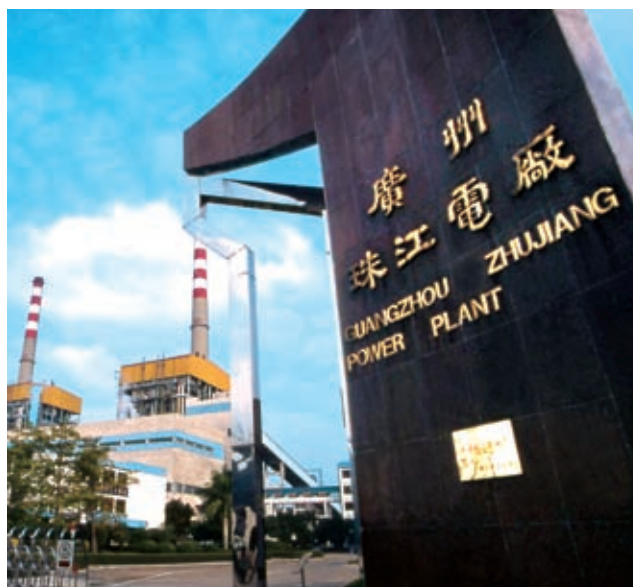
Zhujiang Power Plants
