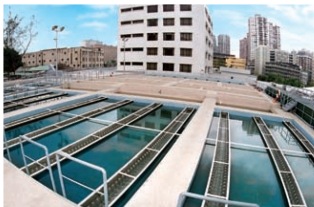
Macau Water Plant
