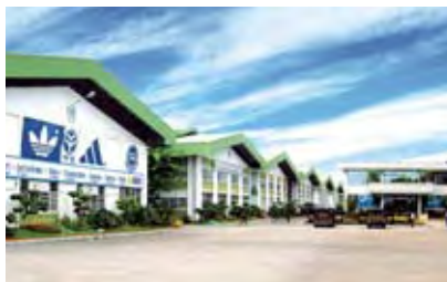
Production facilities in Indonesia
