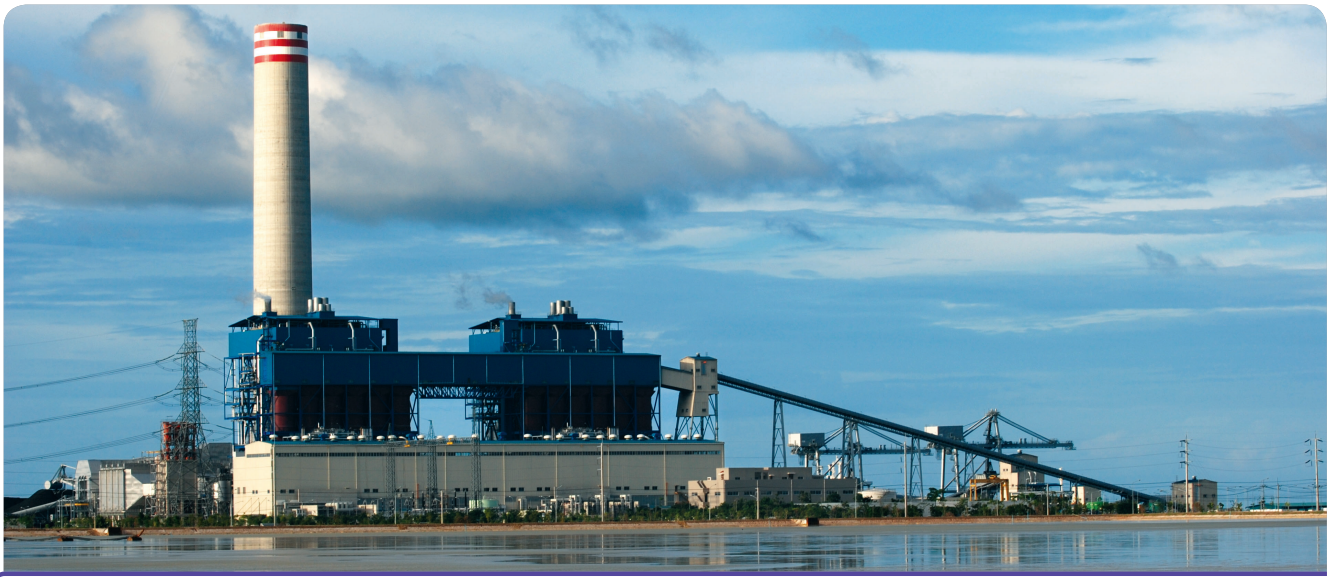
BLCP Power Station
