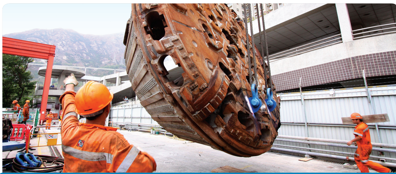
Extracting the cutterhead of the tunnel boring machine at Castle Peak
