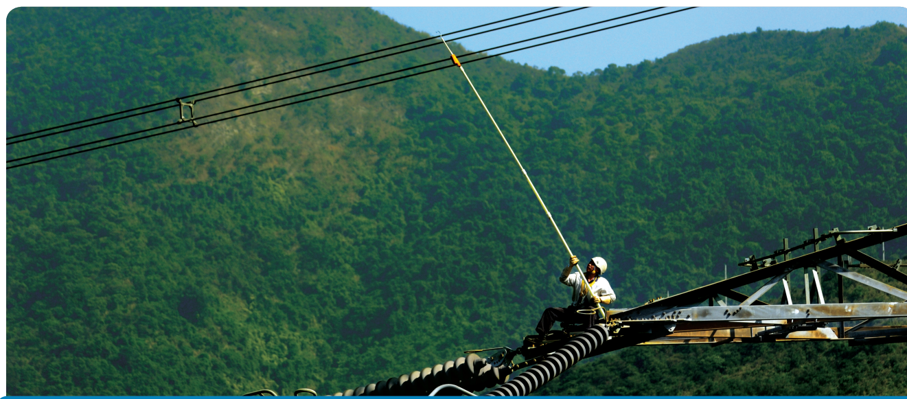
Linesman working on 400kV overhead lines
