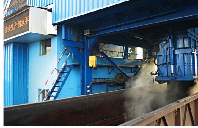
Automatic sealed coal loading system
