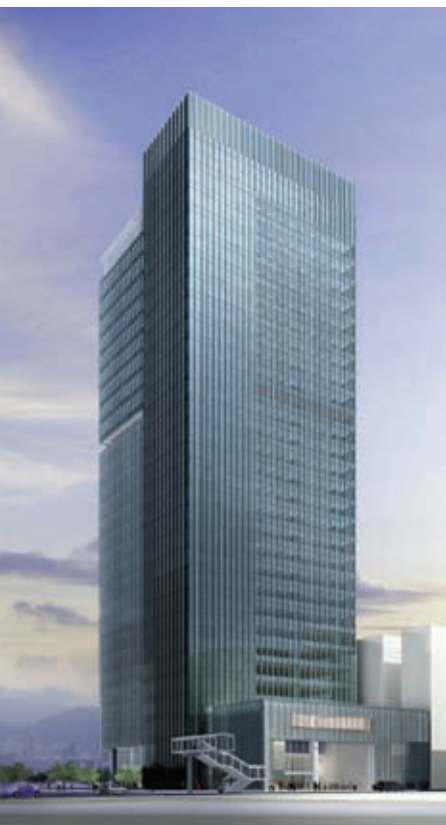
King's Road Project, North Point, HONG KONG*
