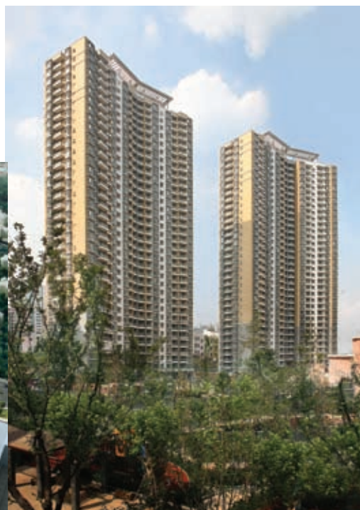
Le Loft, Kerry Everbright City Phase IIB, Shanghai, MAINLAND CHINA
