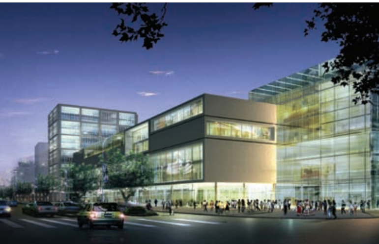
Hangzhou Kerry Centre, Hangzhou, MAINLAND CHINA*
