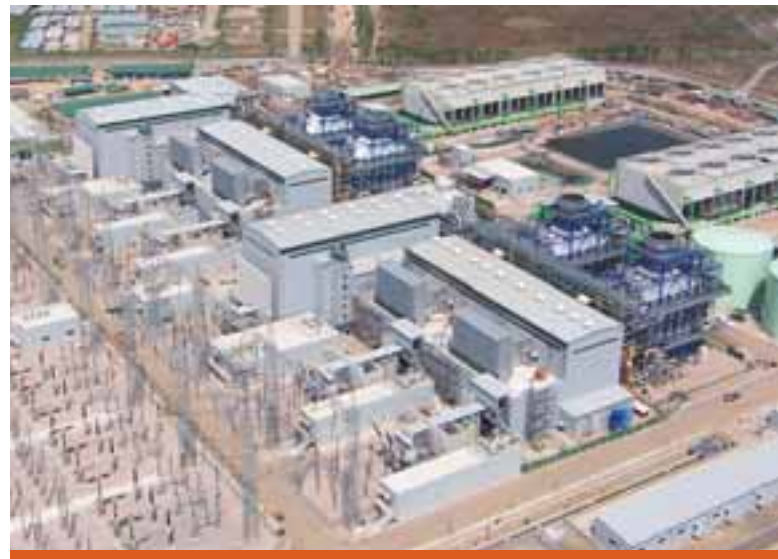
● Commissioned in two phases in March and June 2008 is HEH’s investment in Thailand - Ratchaburi power plant.
