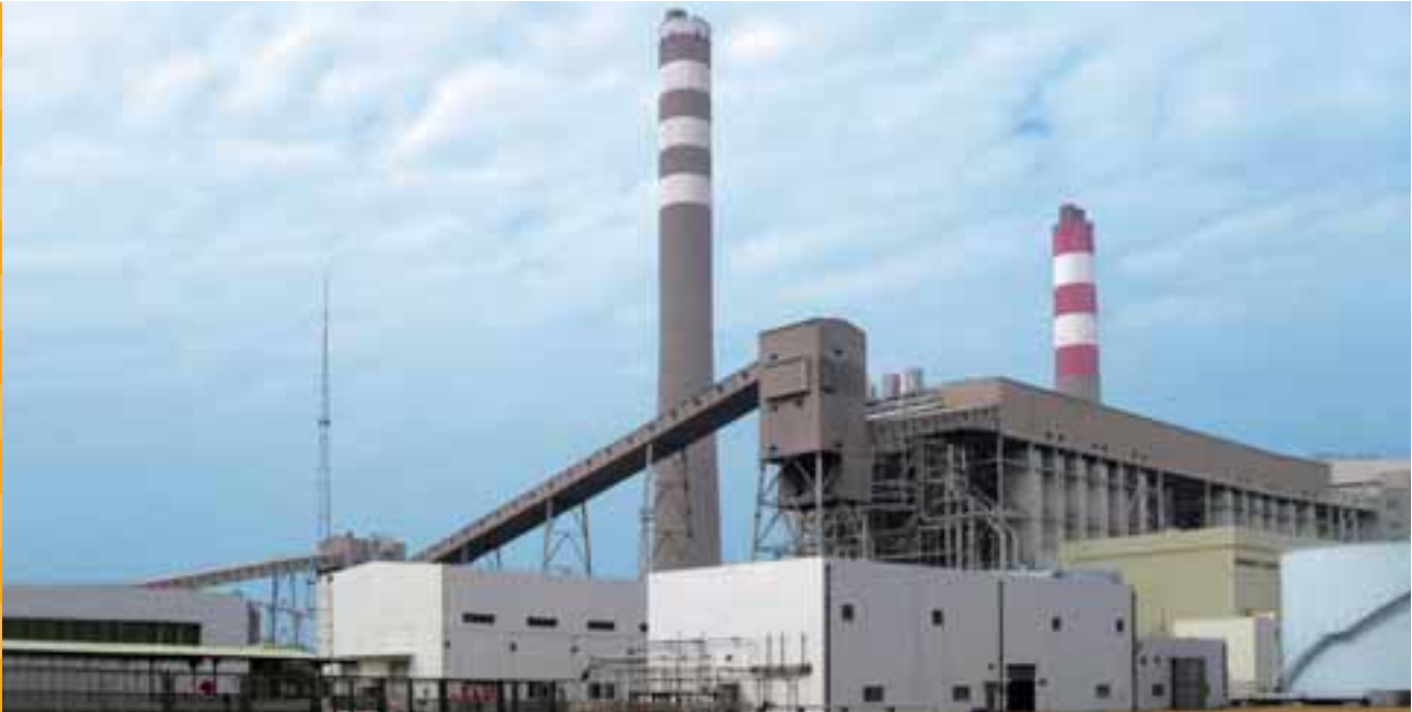
The Zhuhai Power Plant is a very reliable operation with high thermal efficiency.
