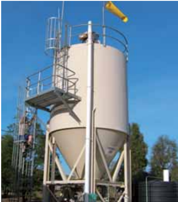
AquaTower is the exclusive potable water supplier for four regional towns in Victoria.
