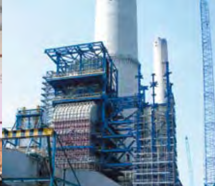
Three Lamma units are being retrofitted with Flue Gas Desulphurisation plants.
