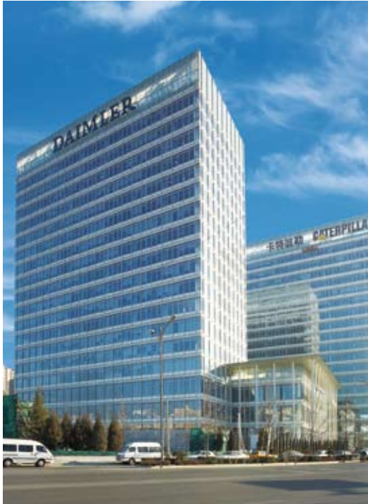
Curtain wall construction by SJQ – Lei Shing Hong, Beijing, the PRC
