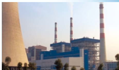
Pingwei Power Plant II
