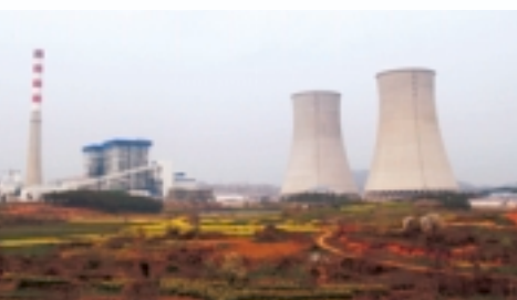
Dabieshan Power Plant
