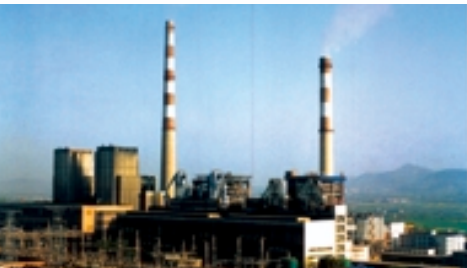
Yaomeng Power Plant
