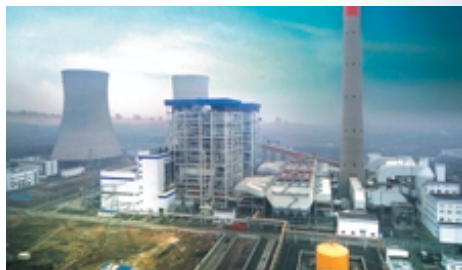
Yaomeng Power Plant II
