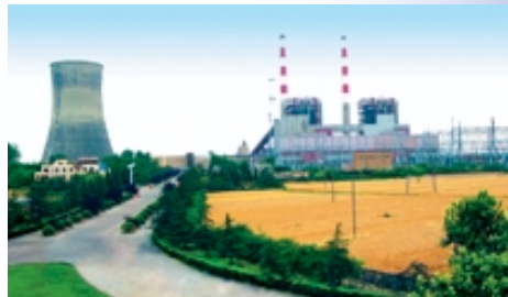
Pingwei Power Plant
