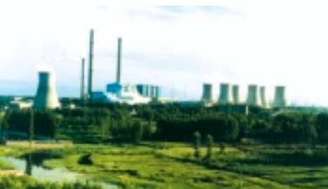
Shentou I Power Plant
