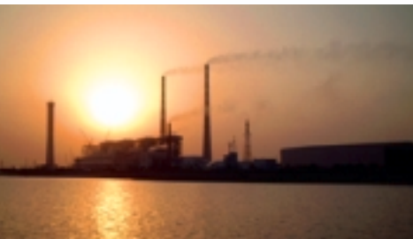
Changshu Power Plant
