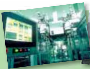
NJCTT's production plant for PVC-free large volume injections
