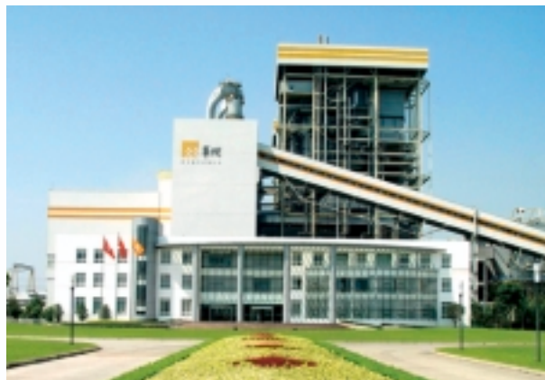
Dengfeng Power Plant
