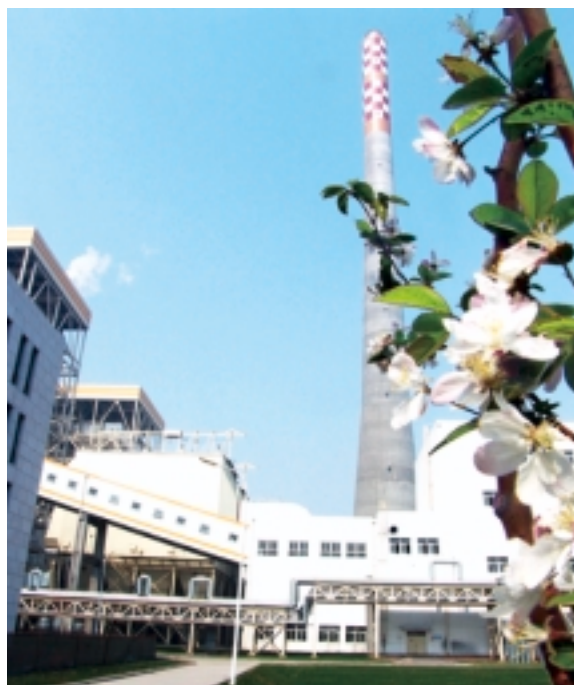
Cangzhou Power Plant
