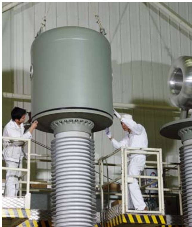
▲ Installation of MWB transformer
