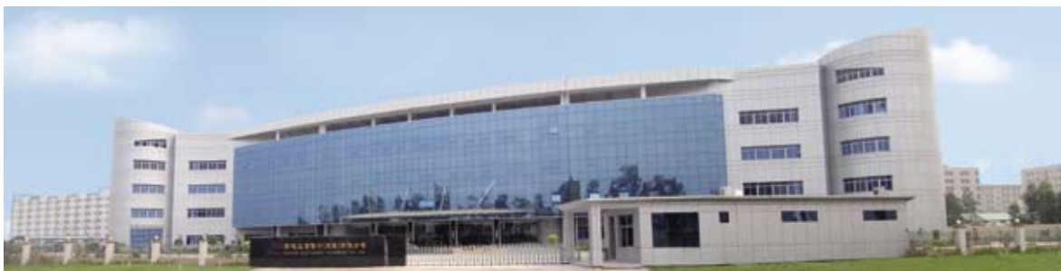
Front view of the Group's E-Caps manufacturing facility located in Changan, Dongguan, PRC
