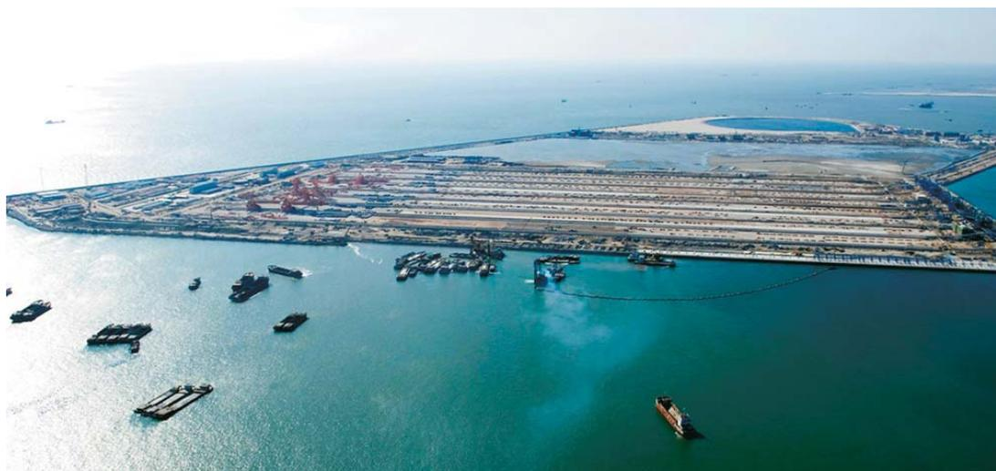
Completion of Basin and Channel dredging of Coal Terminal at Initial Stage in Caofeidian, with dredging volume of 17,400,000 cubic metres
