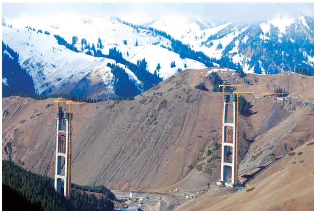
Xinjiang Guozigou Mega Bridge, the first domestic cable-stayed highway bridge with tall tower and steel trussed girder
