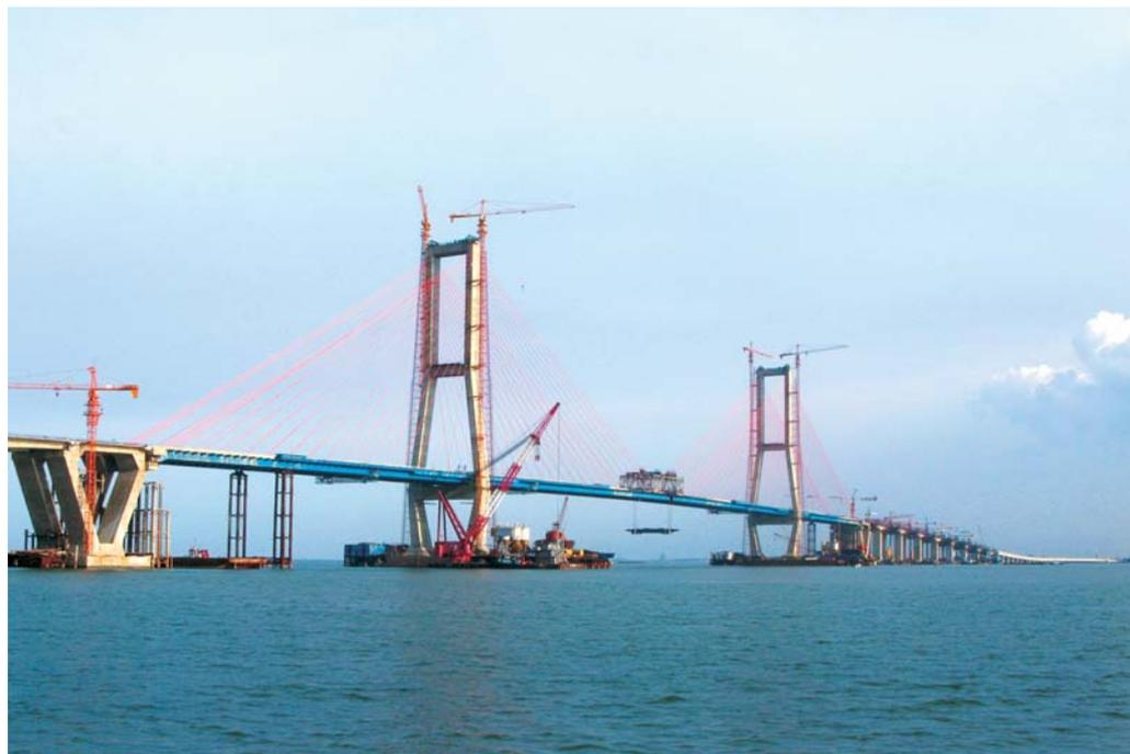
Indonesia Suramadu Bridge with the main bridge of cable-stayed bridge, is expected to be completed in 2009
